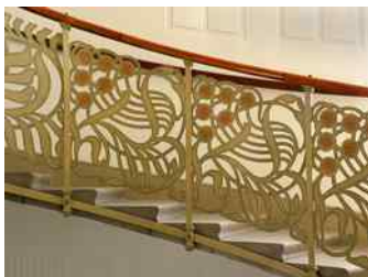
Stairway of the Majolica-Haus (1898)
