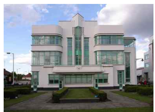
Wallis, Gilbert and Partners The Hoover Building Canteen, Perivale, London 1938
